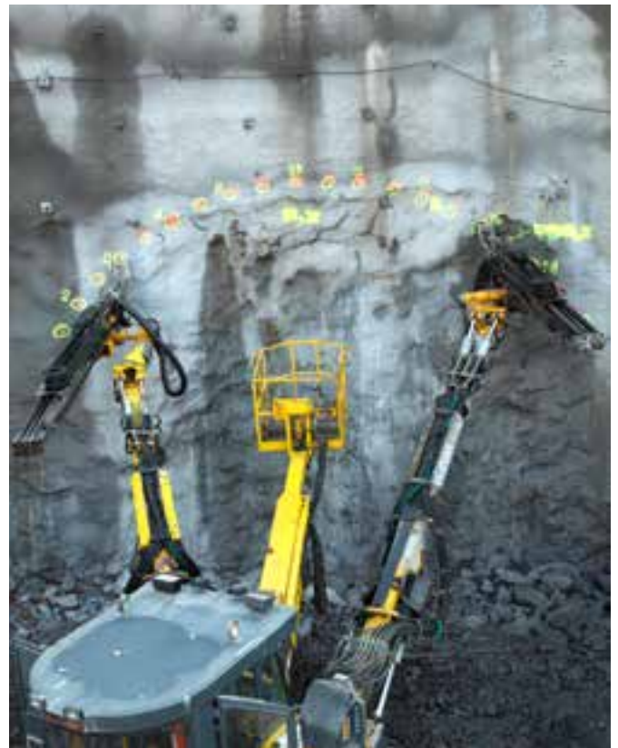
Pipe roofing application with a boomer.
